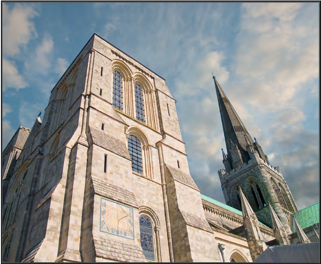
Fig 8.9 the completed image.
