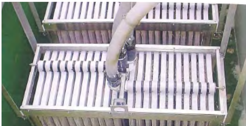
Figure 8.7 module cassettes during In-air cleaning
