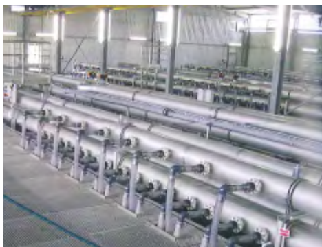
Figure 8.5 membrane installation at the WWTP Nordkanal
