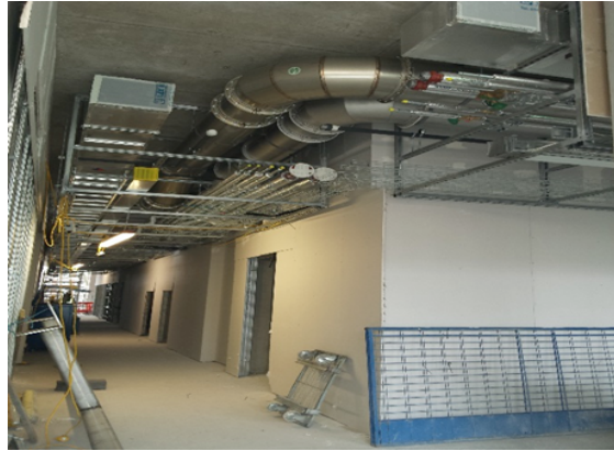
Figure 9.12: An image of the M+E and partitioning installed
